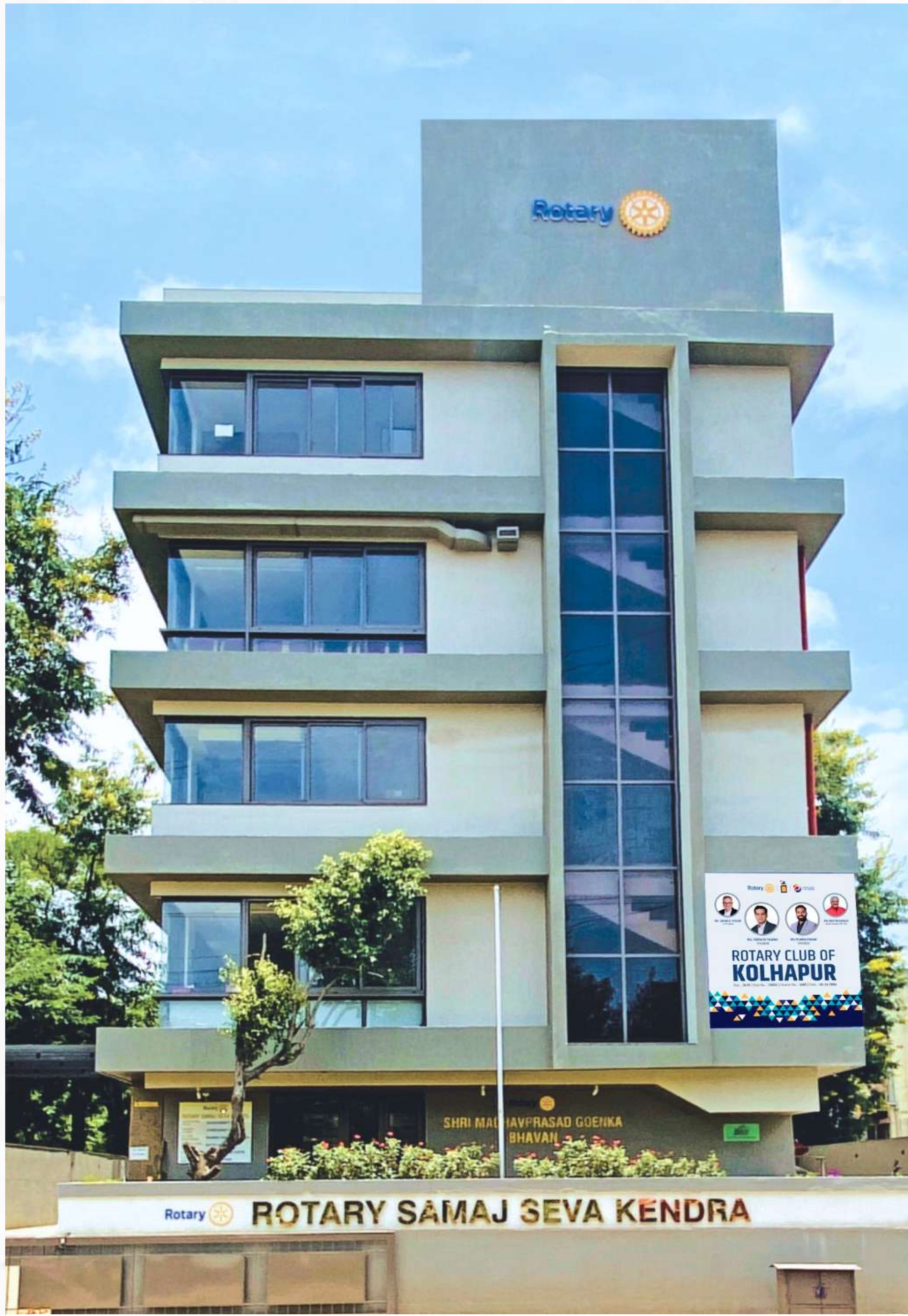
ROTARY CLUB OF KOLHAPUR'S ROTARY SAMAJ SEVA KENDRA BUILDING
